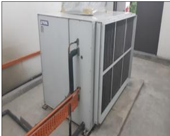
Unit Indoor Sistem ACPU sistem Aircond berkenaan
