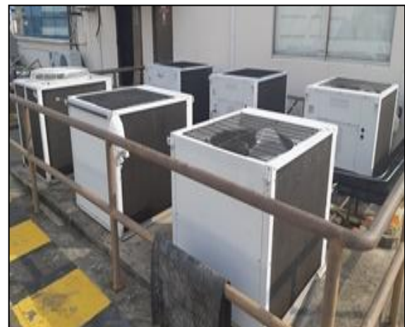
Unit Outdoor Sistem ACPU sistem Aircond berkenaan.
