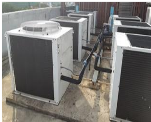
Unit Outdoor Sistem ACPU sistem Aircond berkenaan.
