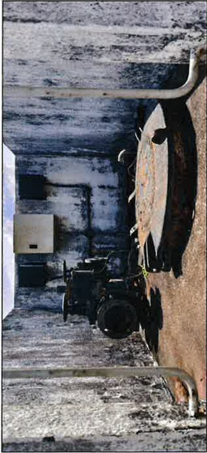
TO REPLACE ISOLATION VALVE, MOTORIZED BREAKER VALVE (AIR INLET VALVE), PIPEWORK, LEVEL ELECTRODE, MANHOLE SEAL, TERMINATION PANEL AND ELECTRICAL WORK.
