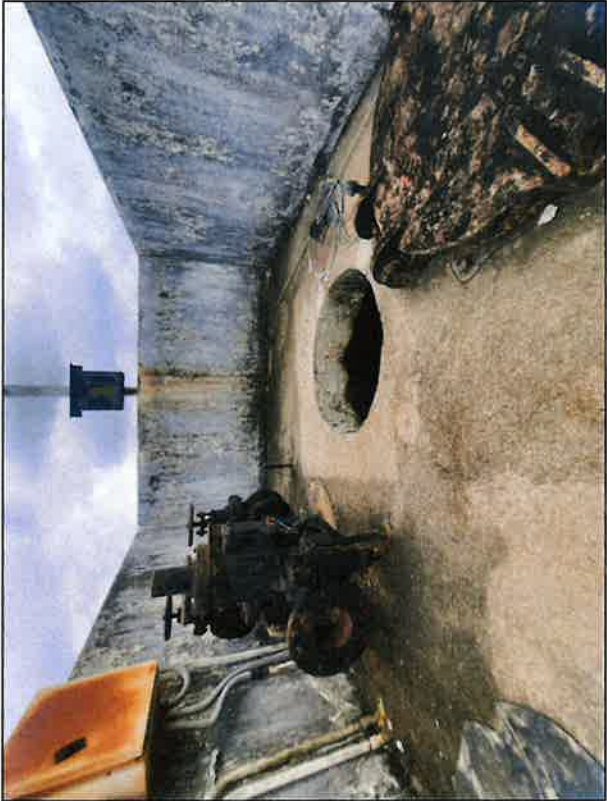
TO CLOSE OPENING AT PULSATOR CLARIFIER NO.1 (PROPOSE TO USE STAINLESS STEEL PLATE)
