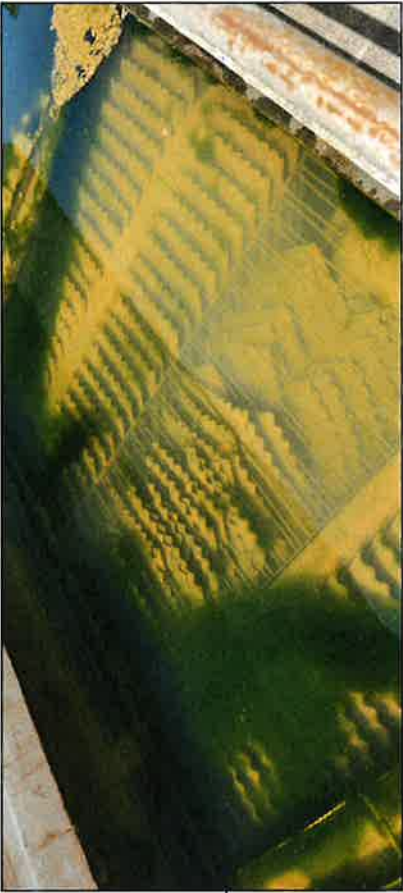
REPLACED EXISTING INCLINED PLATE WITH TUBE SETTLER
