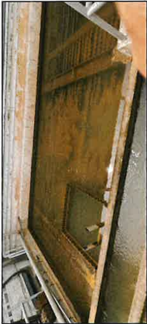
TO REPLACE EXISTING ALUMINIUM LADDER
