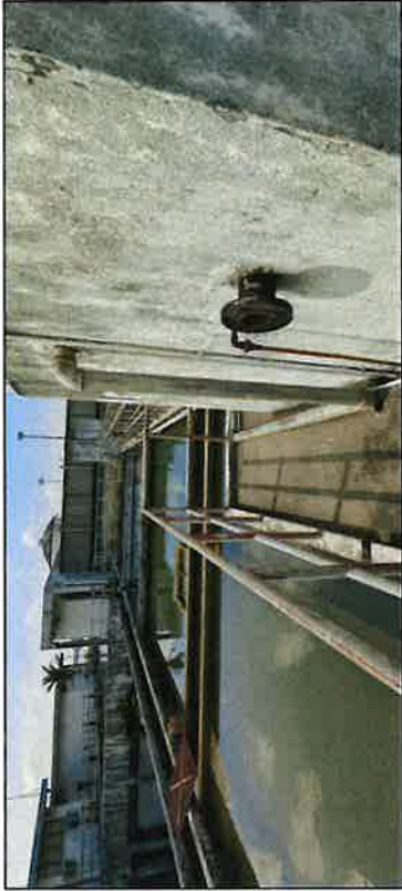
TO REPLACE EXISTING GALVANIZED PIPE FROM VACUUM PUMP
