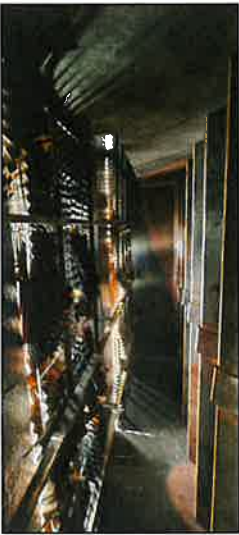
EXISTING INCLINED PLATE AND SUPPORT (VIEW FROM INSIDE PULSATOR CLARIFIER)
