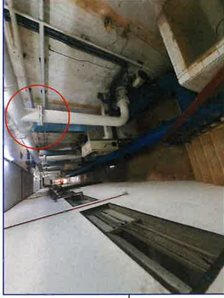
RELOCATION OF THE AIR SCOUR INLET PIPE AND INLET VALVE AS PER TENDERER DESIGN
