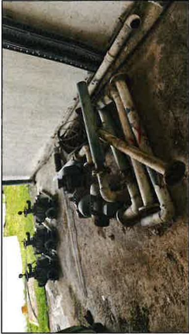
EXISTING VACUUM PUMP AND PIPEWORK (VACUUM SYSTEM NOT IN WORKING CONDITION)
