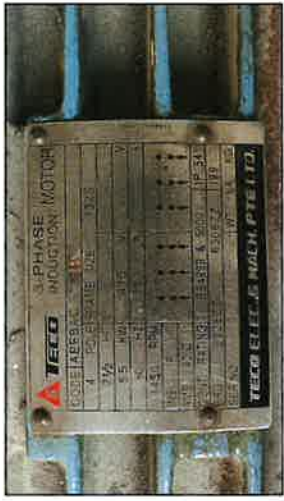
EXISTING VACUUM PUMP MOTOR DATA
