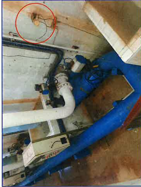
REPLACE FILTER LOSS OF HEAD INSTRUMENT
